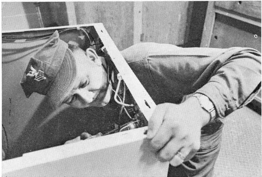
There's a giant in this washer—CE1 Sam Teare, who is getting the machine back in service for a base family.
