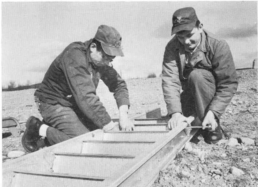
Installing recreation equipment at the new school are EN1(SS) Marshal Chapman and EN1(SS) Dale Byrd.
