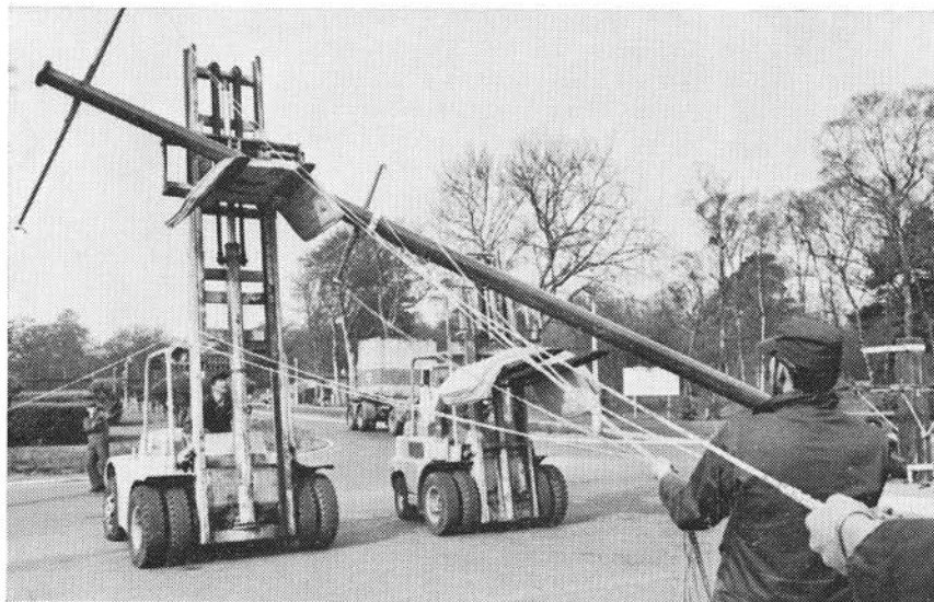
Two forklifts were used to slowly lower the pole and keep it from being damaged.
